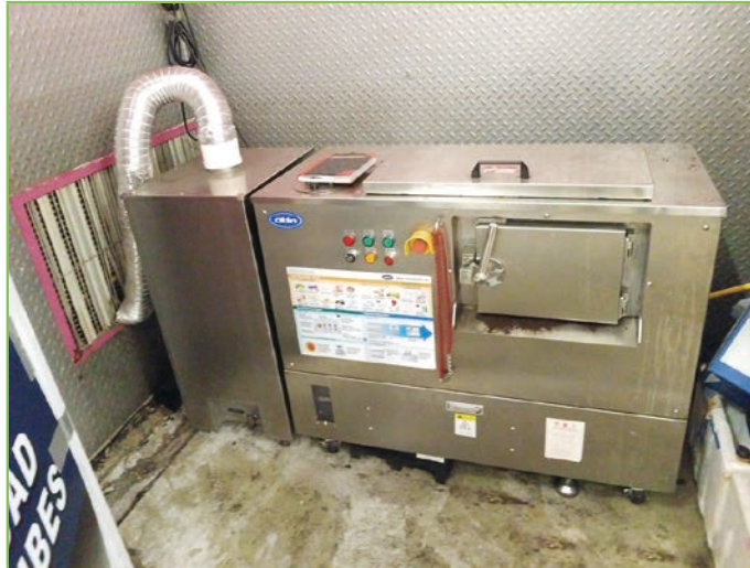
The food waste recycling machine in The ONE. 設置在The ONE內的廚餘回收機。
